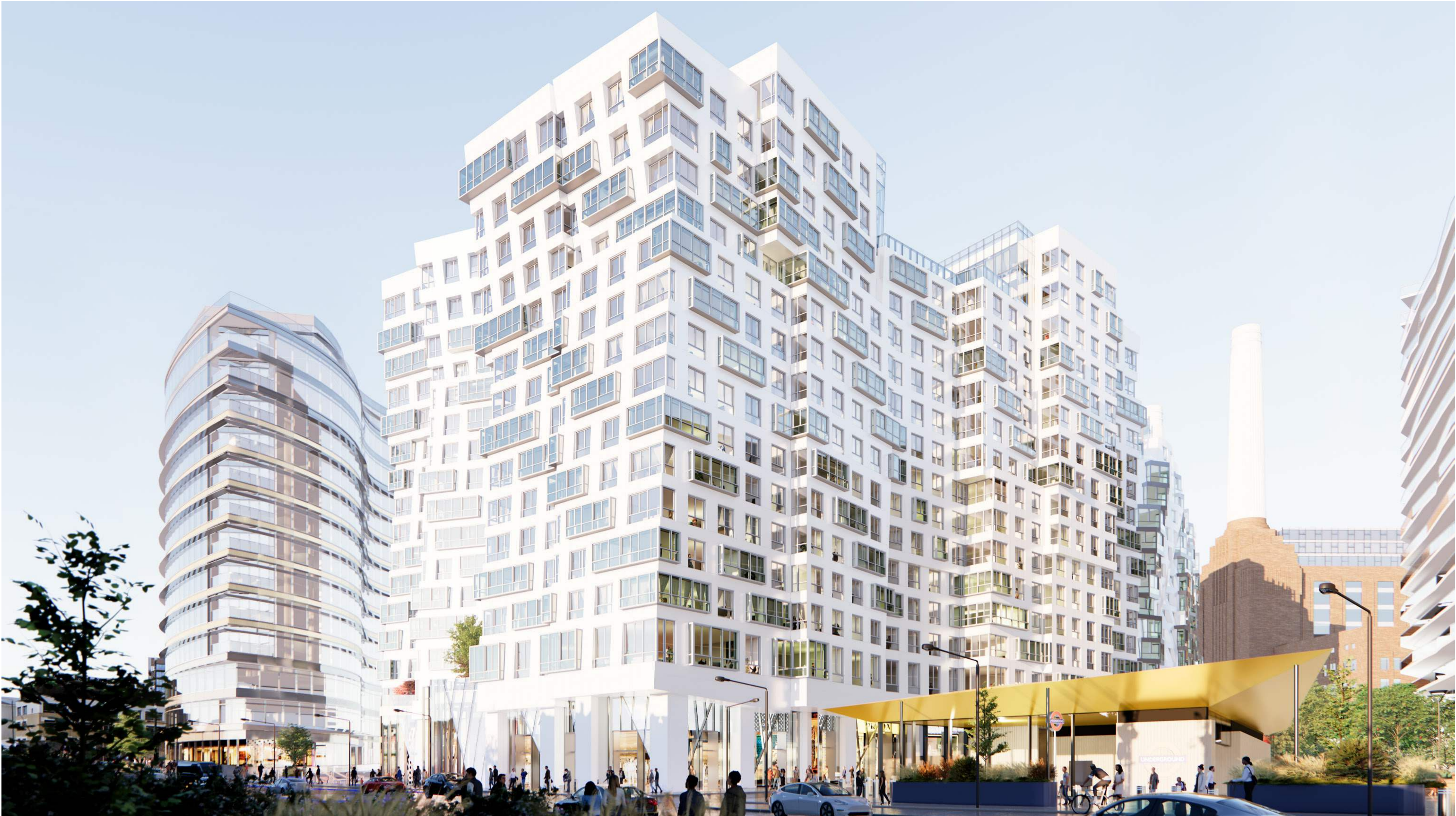
VIEW FROM SOUTHERN SIDE OF BATTERSEA PARK ROAD LOOKING WEST
